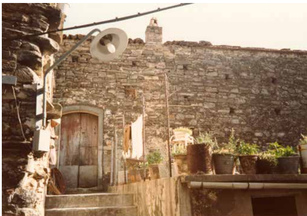
Fig. 6: Example of a traditional house built with Cirigliano stone (1980s).
