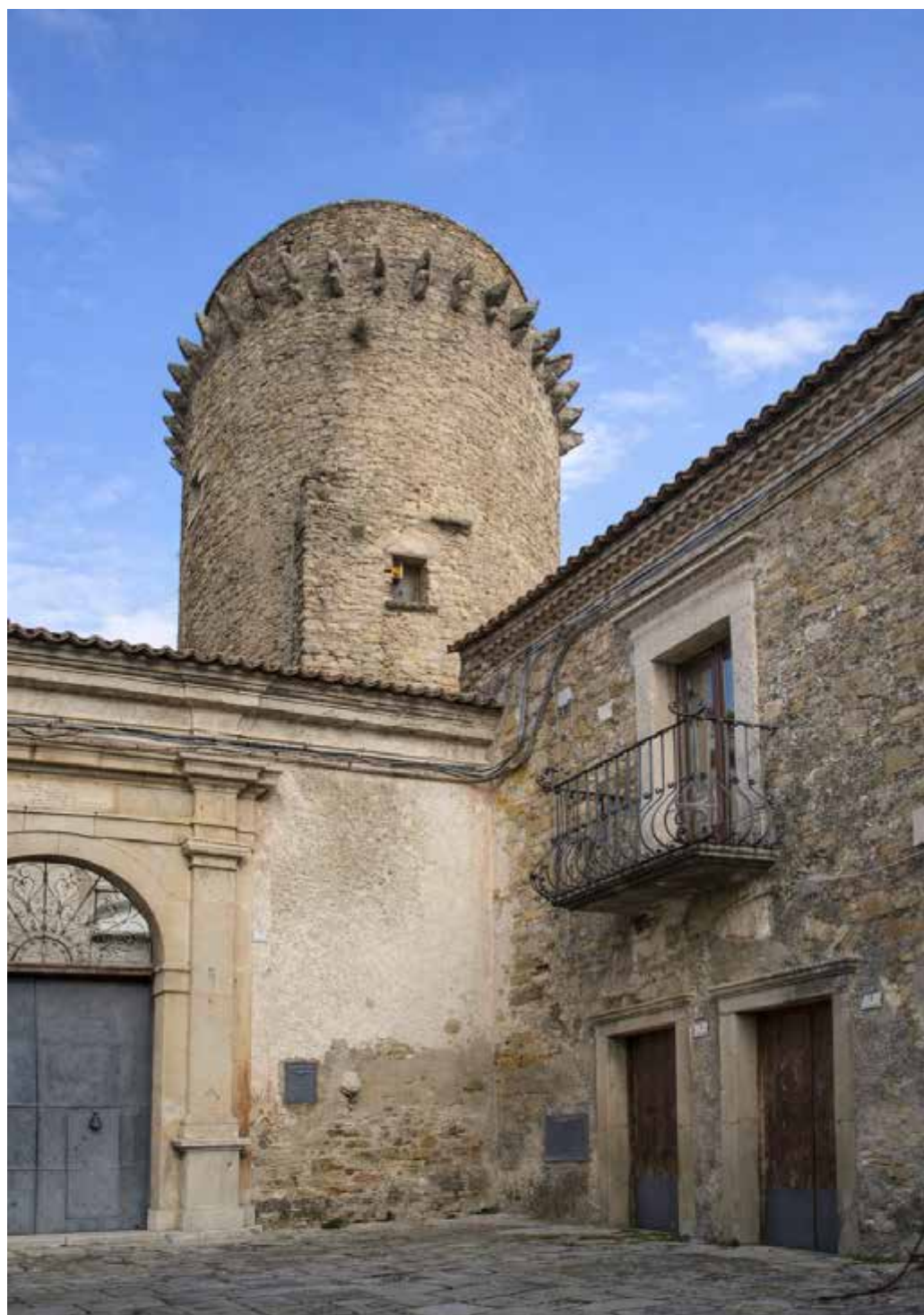
Fig. 15: The entrance portal of the castle and its tower.
